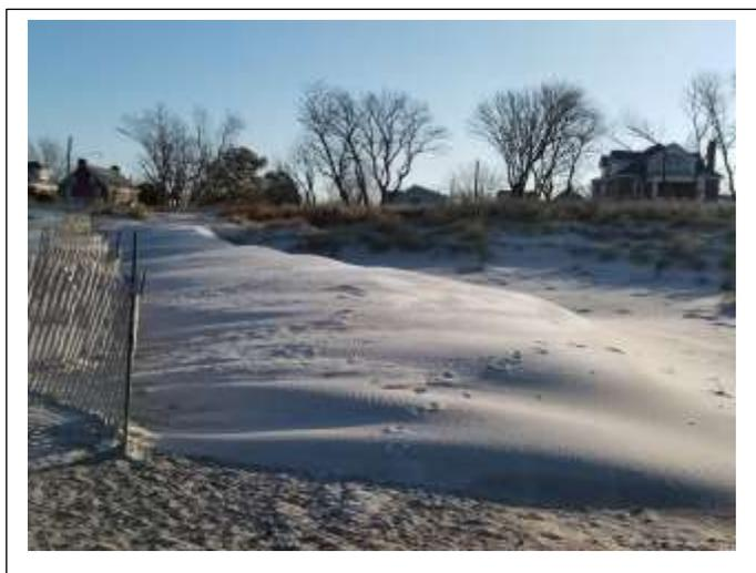
**Figure 9.** Temporary sand fences at Madison Ave. trapping blowing sand (A.H. Walker photo)
