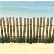
The Public Works crew will be closing the Jefferson Avenue beach access today using erosion fence and burlap. This is the worst area where sand blows onto Bay Avenue. There is very little beach to sidewalk ratio in this area and no grass to help hold the sand. The new fence will help build up the sand in this area. A temporary wooden post will also be installed with safety rope fencing along the edge of the sidewalk due to the drop-off in this area.
